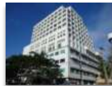
Siloam Hospitals Manado and Hotel Aryaduta Manado
