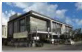
Siloam Hospitals Bali
