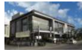
Siloam Hospitals Bali
