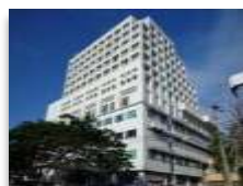
Siloam Hospitals Manado and Hotel Aryaduta Manado
