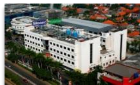
Siloam Hospitals Kebon Jeruk
