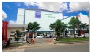
Siloam Hospitals Purwakarta
