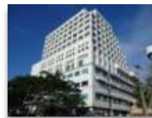
Siloam Hospitals Manado and Hotel Aryaduta Manado
