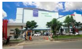
Siloam Hospitals Purwakarta
