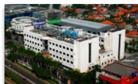
Siloam Hospitals Kebon Jeruk
