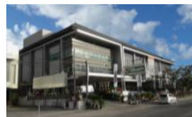
Siloam Hospitals Bali
