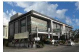
Siloam Hospitals Bali
