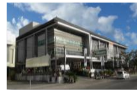
Siloam Hospitals Bali
