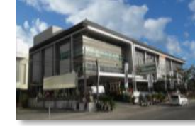
Siloam Hospitals Bali
