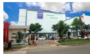
Siloam Hospitals Purwakarta
