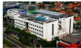
Siloam Hospitals Kebon Jeruk
