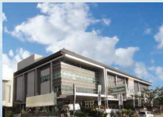
Siloam Hospitals Bali
