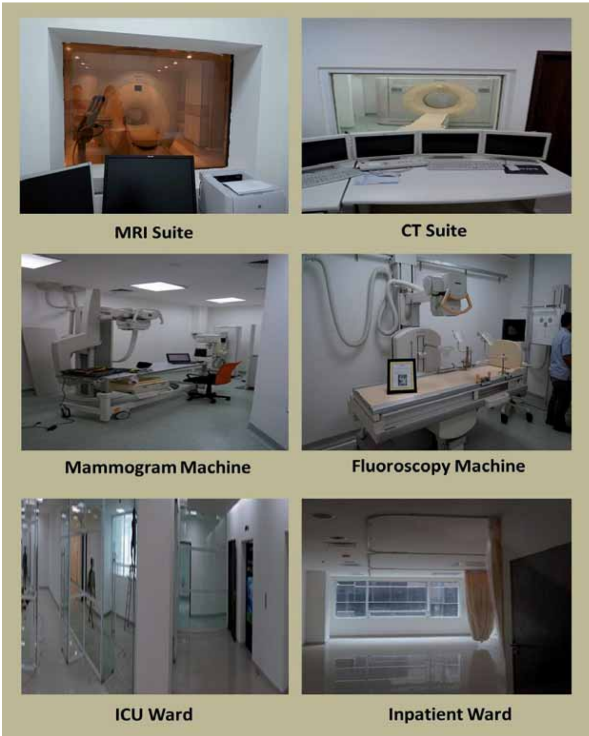
Figure 3.9: Current completed sections and installed equipment at SHMD (cont)
