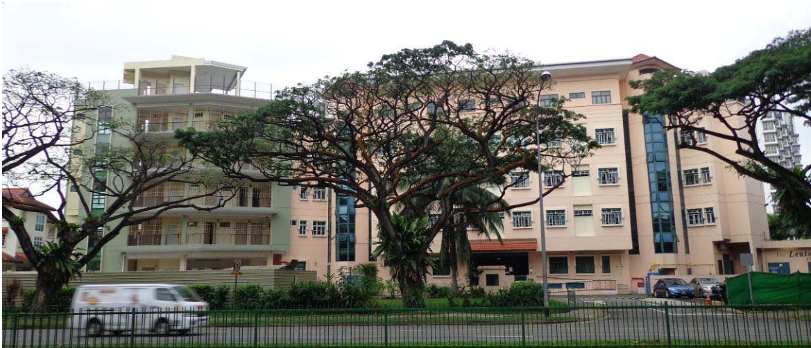
Photo of Extension Building and Existing Building
