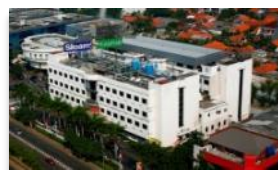
Siloam Hospitals Kebon Jeruk
