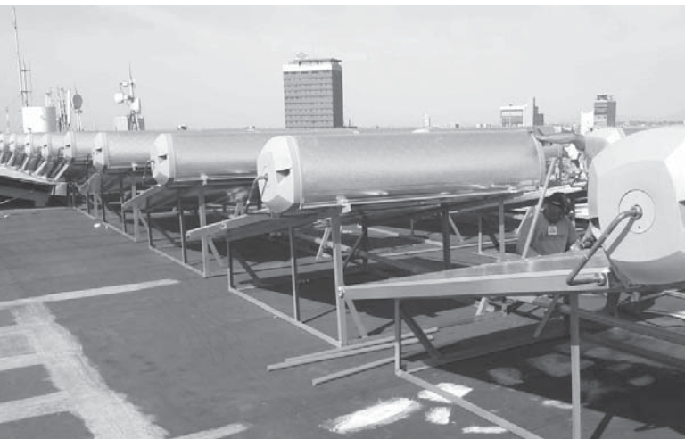
Installed Solar Panels on SHMK rooftop
