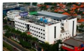
Siloam Hospitals Kebon Jeruk
