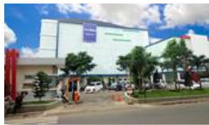
Siloam Hospitals Purwakarta
