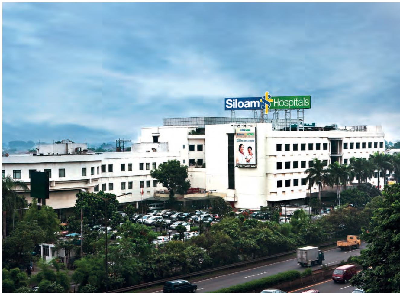
Siloam Hospitals Kebon Jeruk
