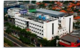
Siloam Hospitals Kebon Jeruk
