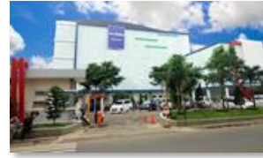
Siloam Hospitals Purwakarta
