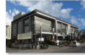
Siloam Hospitals Bali
