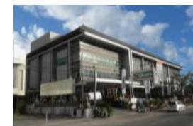
Siloam Hospitals Bali
