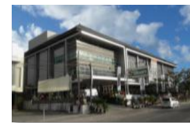
Siloam Hospitals Bali
