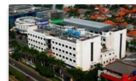
Siloam Hospitals Kebon Jeruk
