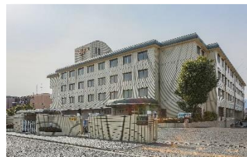
ElySION Mamigaoka & Annex
